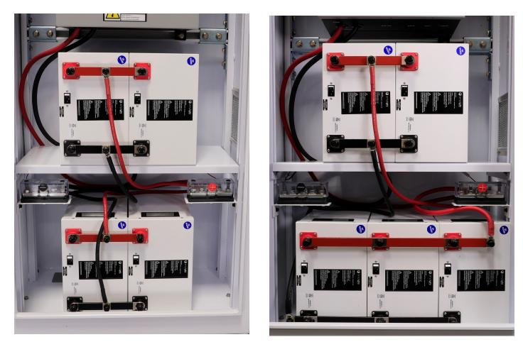
Figure 11.0a-Four PHI Battery Orientation
