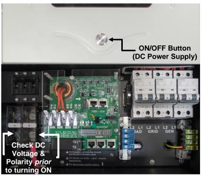
Figure 18.0 – Inverter & DC Power Supply ON/OFF Button
