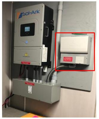
Figure 7.0 – Transfer Switch Kit
